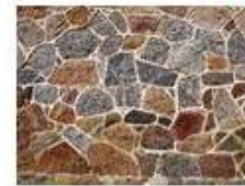
compound wall with stone masonry
