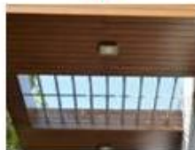
fundermax under roof cladding
