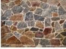
compound wall with stone masonry
