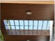
fundermax under roof cladding
